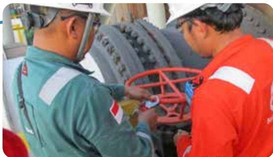
Proses Pemasangan Log Out – Tag Out (LO-TO) di Cooling Water Area
