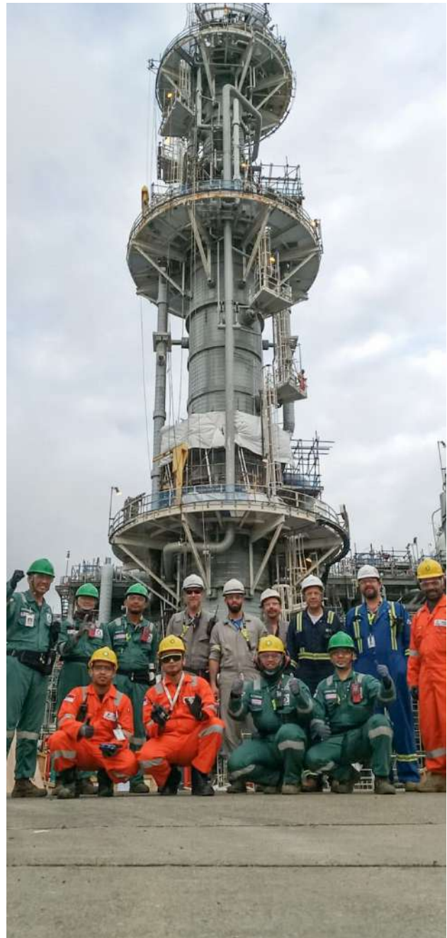
● Badak LNG employee involved in the MCHE repair project at Tangguh LNG
