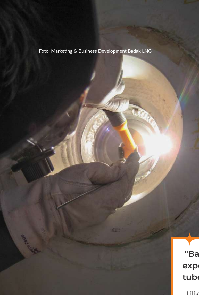
📍 Tube welding activity during the MCHC repair work at Yemen LNG
