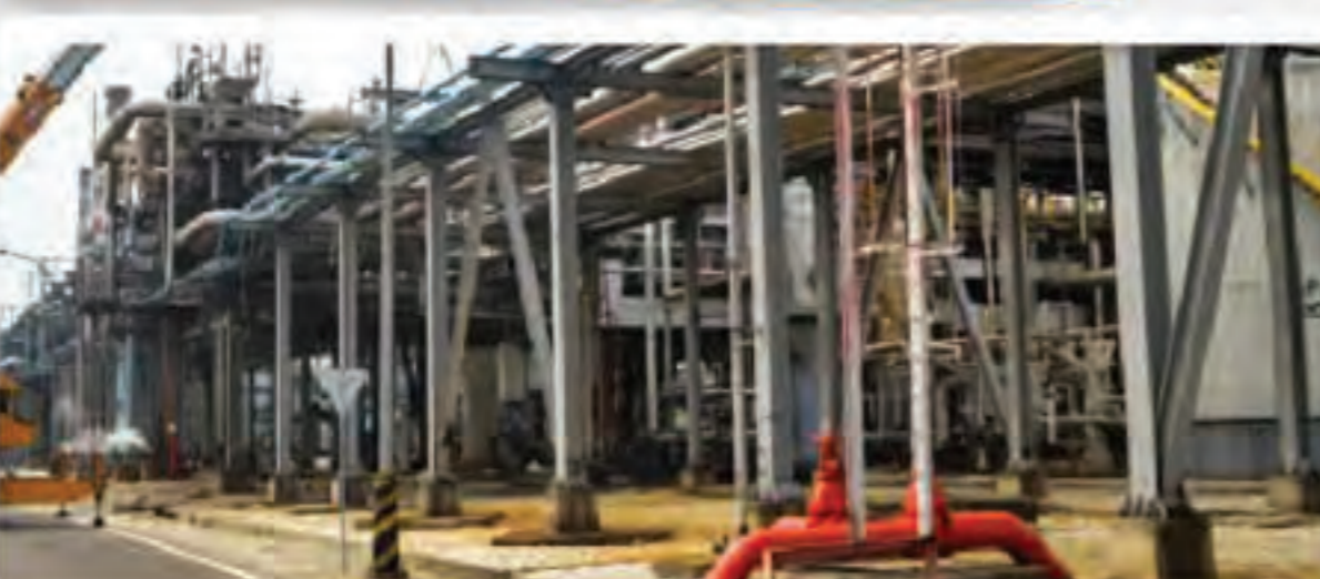
Pengangkatan material di process train area .
