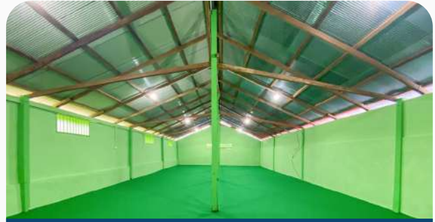
Ruangan lantai 2 setelah direnovasi 2 nd floor room before renovation
