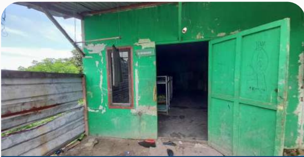
Tampak depan sebelum direnovasi Front view before renovation
