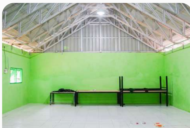
Tampak Gedung serbaguna setelah direnovasi Multipurpose building after renovation
