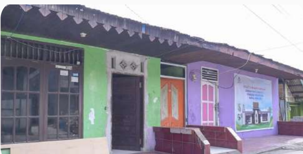
Tampak depan sebelum renovasi Front view before renovation
