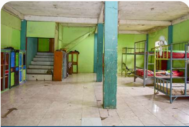
Kamar santri sebelum direnovasi Student room before renovation
