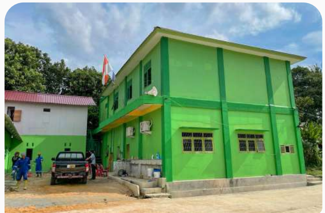
Tampak belakang sesudah direnovasi Rear view after renovation
