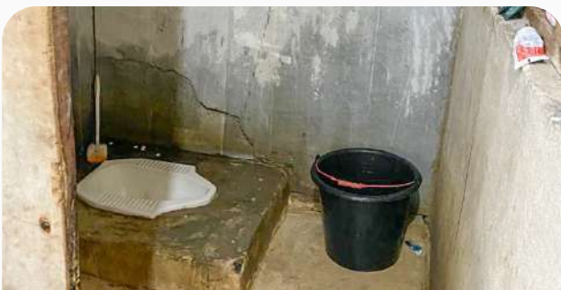
Toilet sebelum direnovasi Toilet before renovation
