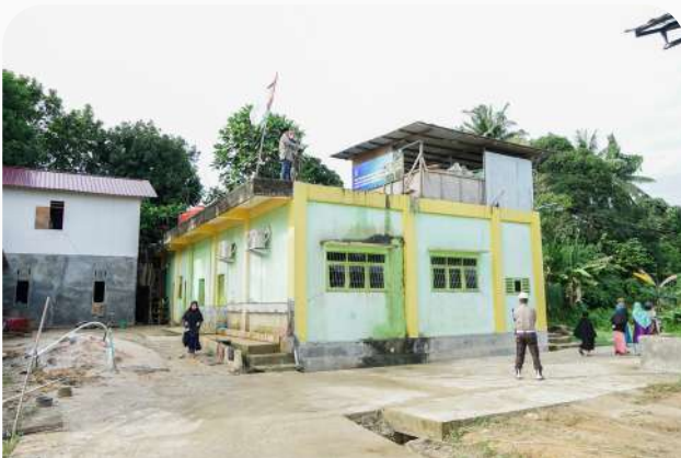
Tampak belakang sebelum direnovasi Rear view before renovation
