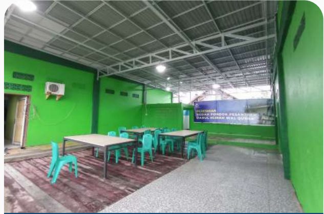
Tempat wudhu sesudah direnovasi The ablution facility after renovation
