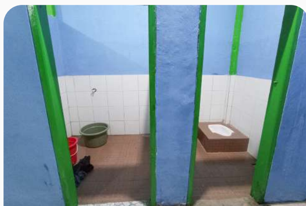
Toilet setelah direnovasi Toilet after renovation
