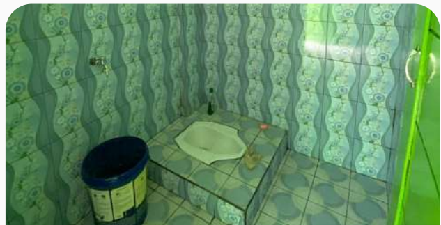
Toilet setelah direnovasi Toilet after renovation
