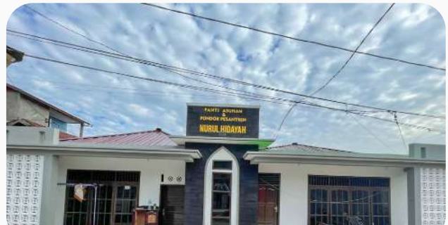
Tampak depan setelah renovasi Front view after renovation
