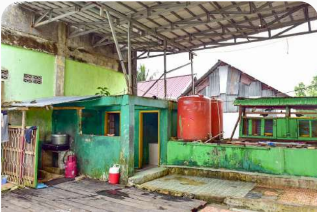
Tempat wudhu sebelum direnovasi The ablution facility before renovation
