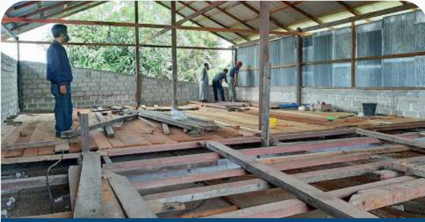
Ruangan lantai 2 sebelum direnovasi 2 nd floor room before renovation
