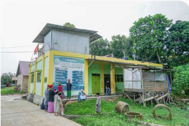
Tampak depan sebelum direnovasi Front view before renovation
