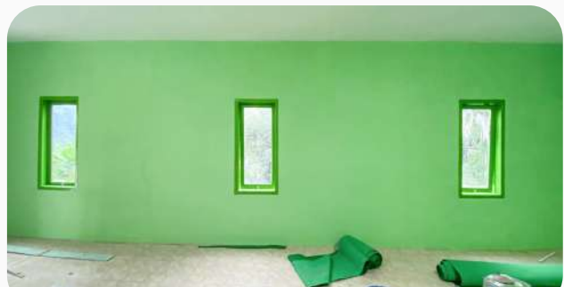
Kamar tidur santri setelah direnovasi Student bedroom after renovation
