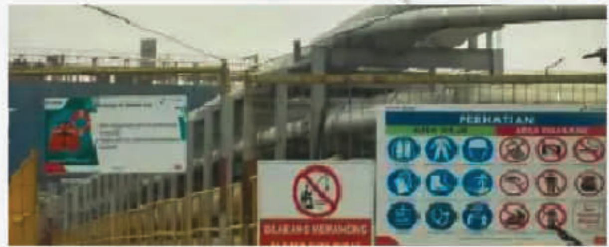
Memasang safety board di area ring of fire atau zone-1 ( high risk area ).
