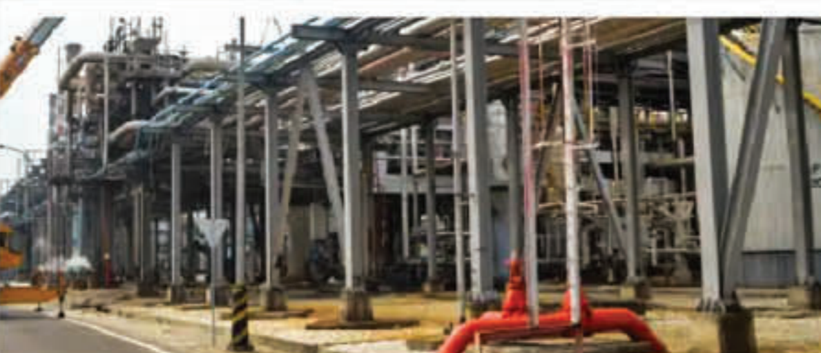
Pengangkatan material di process train area .
